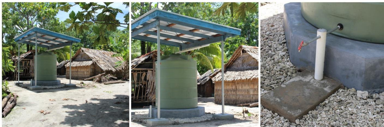
One of the rainwater harvesting systems installed under the project
